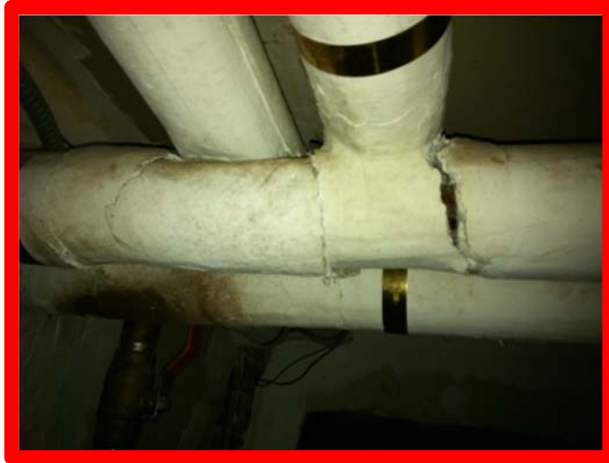
Suspicious pipe insulation may contain asbestos
