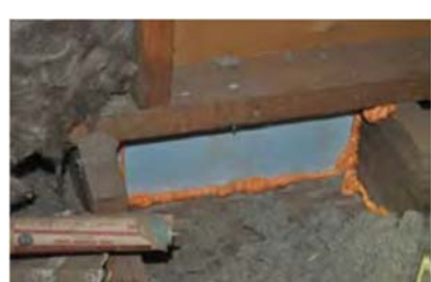
Bottom plate is also sealed to surrounding joist and framing
