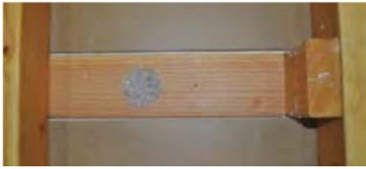
Option 1: Dense pack cavities through wood cap fastened in place
