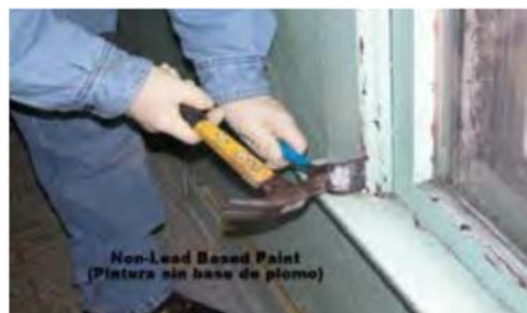
2. Remove stop moulding (non-lead based paint). For lead based paint work requirements, visit http://www2.epa.gov/lead
