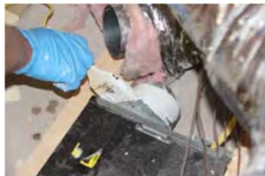
Apply mastic to fan connection
