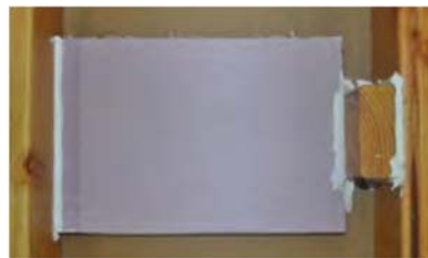
Option 3, Step 2, Option A: Cap with XPS and seal exposed joints
