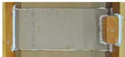
Option 3, Step 2, Option B: Cap with drywall and seal exposed joints
