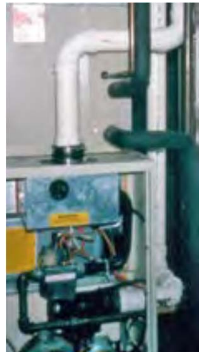
Two-pipe 90% efficiency furnace
