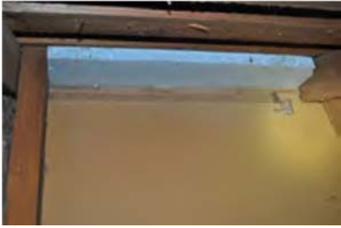
Top plate has been cut and fit to size
