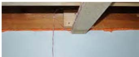
Apply appropriate sealant dependent upon size of crack and location
