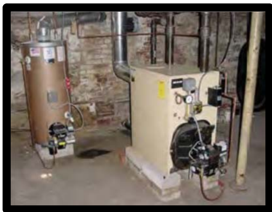
Check oil-fired furnaces and water heaters for proper fuel pressure
