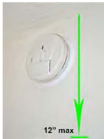
Wall mounted smoke alarms must be mounted within 12 inches of the ceiling
