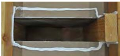
Option 3, Step 1: Apply sealant around opening and on surrounding framing
