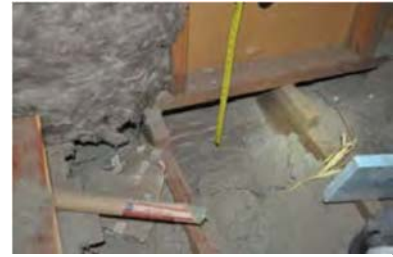
Bottom plate is also missing. Space is measured so XPS can be cut
