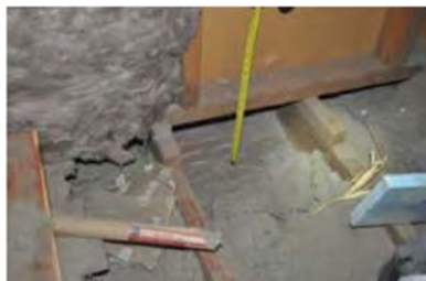
Measure floor cavity for new blocking
