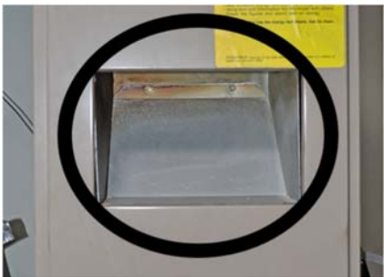
Category I 70% efficiency gas furnace with intake vent circled
