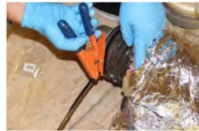
Use zip tie and tensioner to secure liner to connection fitting
