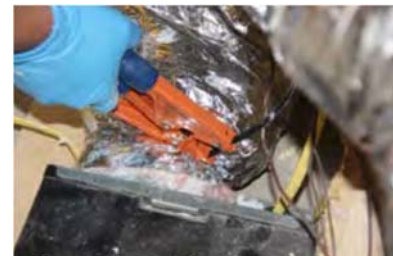
Snug insulation to fan housing and strap into place
