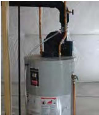
Power-vented water heater
