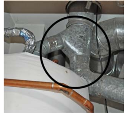
Common vent of natural draft appliances highlighted
