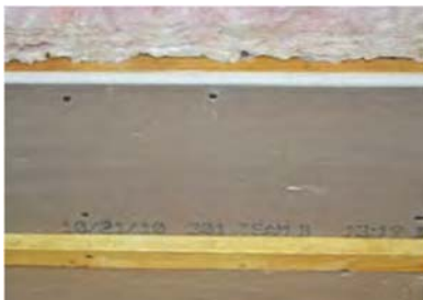
Option 3: Stud bay will faced with rigid material, fastened and sealed
