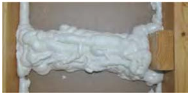
Option 2: Bridge cavities with spray foam
