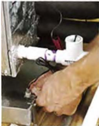
Float switches should be installed in drainage pans to prevent overflow
