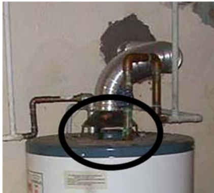
A stand alone natural draft water heater
