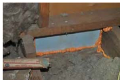
Air seal around new blocking with spray foam
