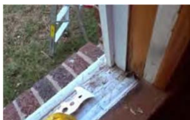
4. Scrape loose paint and thoroughly clean opening.
