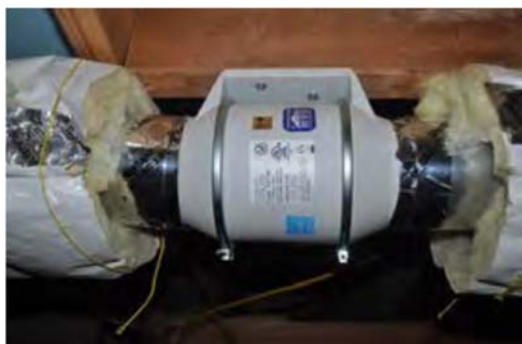
Appliance exhaust, such as that for a dryer, can cause depressurization
