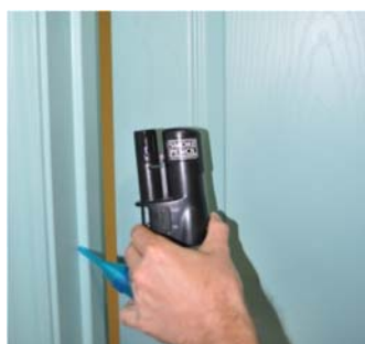
7. Check interior doors for pressure differential either using smoke pencil or hand
