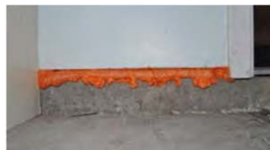
Ensure sealant does not decrease wall's fire resistance
