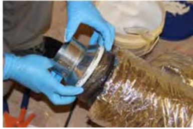
Snug duct liner onto connection fitting
