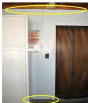
Inspect wall and ceiling for cracks and penetrations
