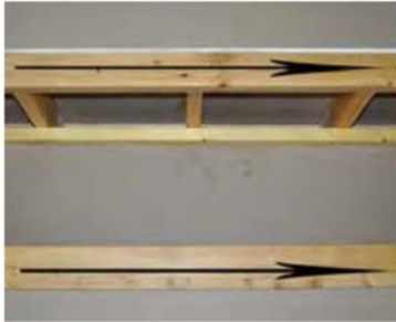
Option 1, Step 1: Apply sealant to top plates or other relevant surfaces
