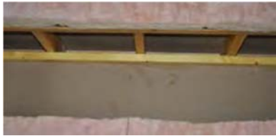
Clear work area of insulation and debris
