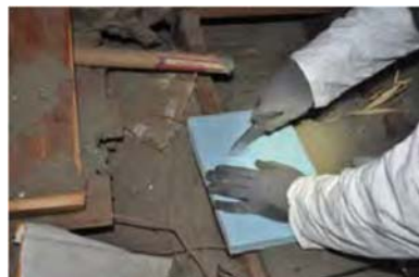
Cut rigid material, such as XPS, to size to snugly fit into cavity
