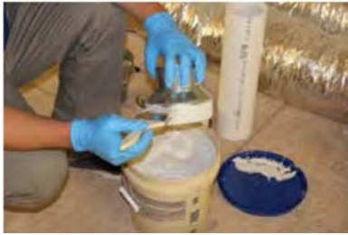
Apply mastic to the connection fitting
