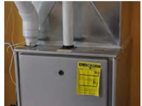
Two-pipe 90% efficiency furnace
